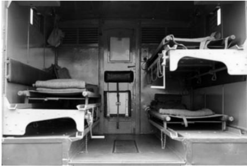
Fig 7.2a - The rear body, built by Mann Egerton, could take 10 casualties sitting or 4 stretcher cases.
